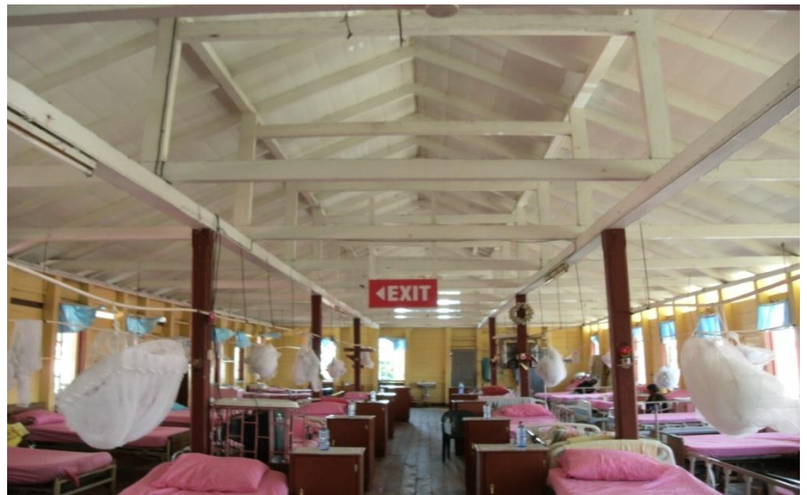
Fig. 2 – Refurbished Ward 8. (photographed 8/10/2015)
